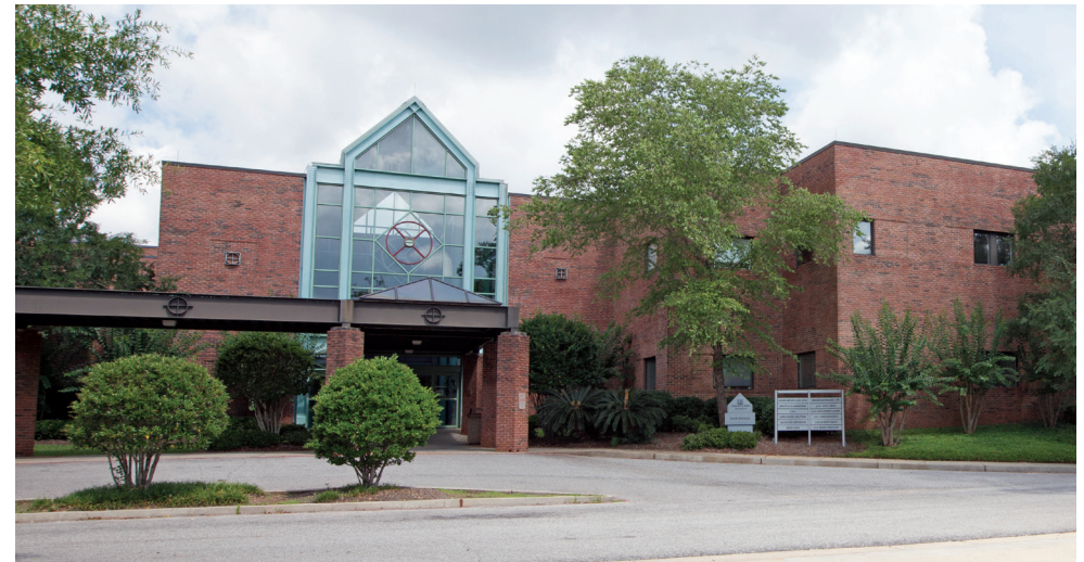
USA Technology & Research Park, Building III
